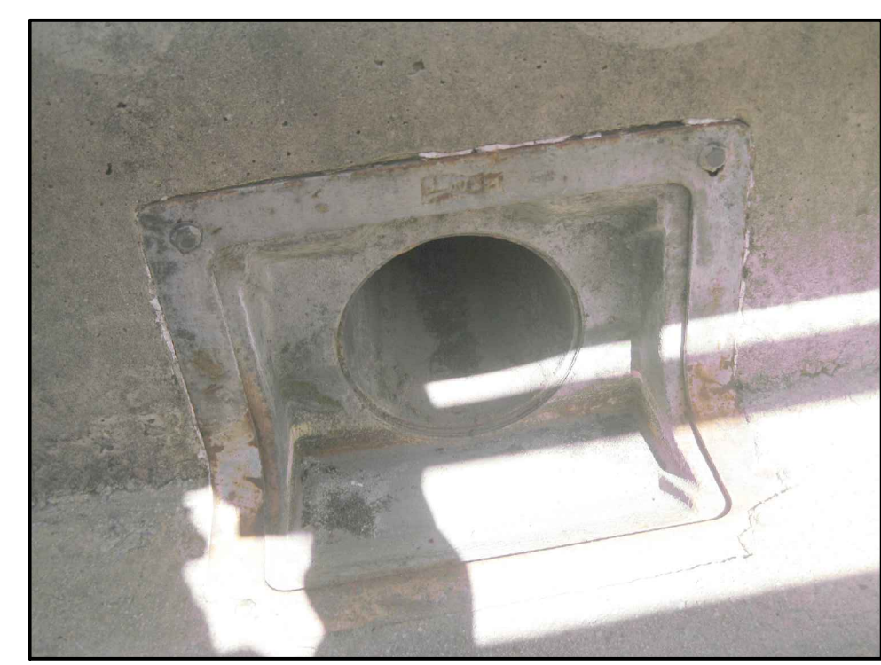
11a EXISTING FLOOR DRAIN
