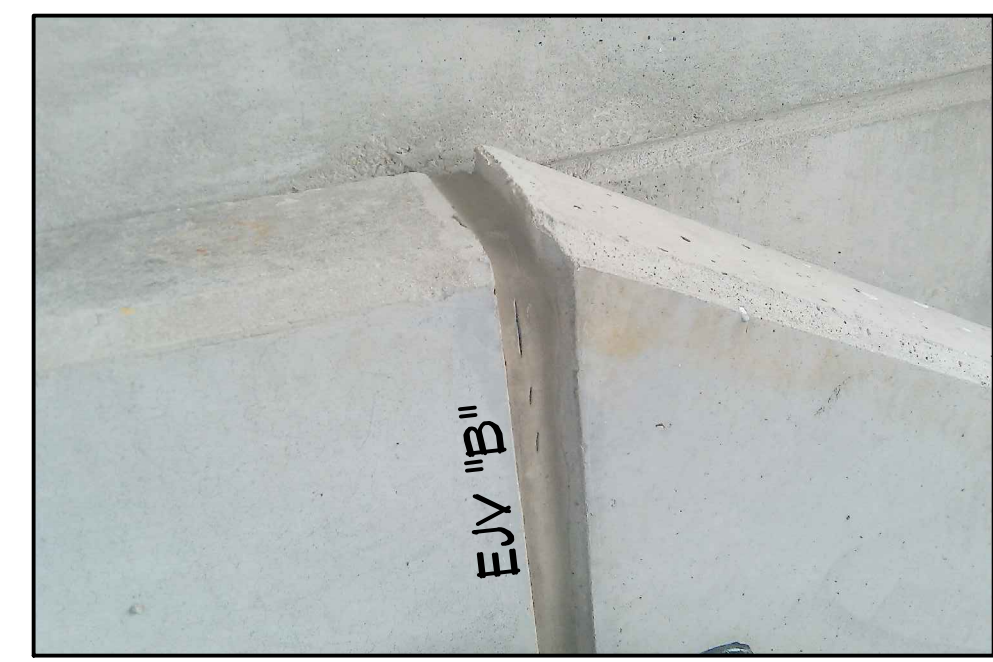
2 VOMITORY WALL VERTICAL JOINT, TYPICAL.
