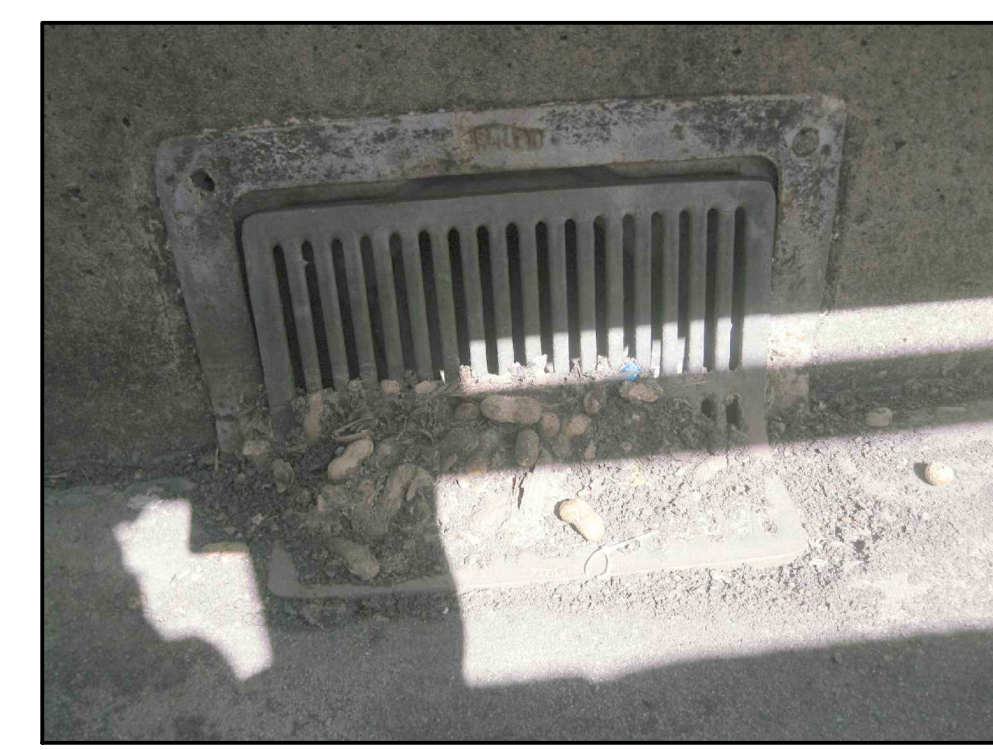
11b EXISTING FLOOR DRAIN (W/ COVER)
