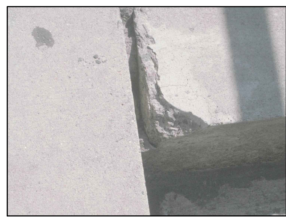
10b MISCELLANEOUS EXAMPLES OF CONCRETE REPAIRS
