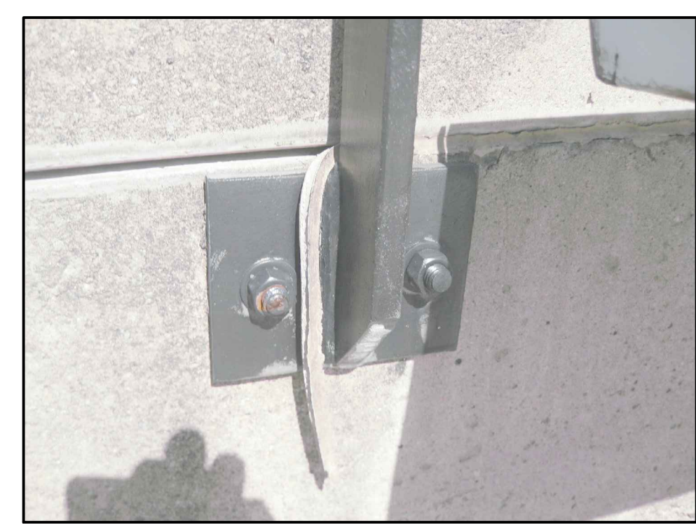
14b VOMITORY RAILINGS MOUNTS
